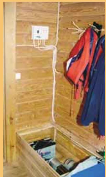
200-W fuel cell battery connected to the solar panel system of a summer cottage. The fuel cell battery will secure electricity in the spring and autumn.
